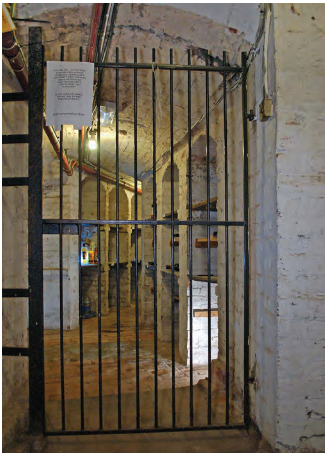
Barred gate to bayed and alcoved bottle store – and considerably more tunnel space than initially appears
